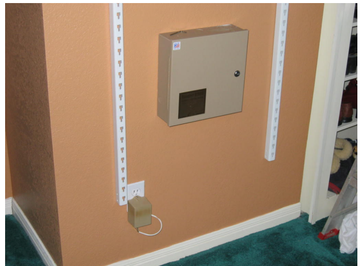
Short Wall trimmed 48" top rail, verticals & shelves adjusted to go around obstacles
