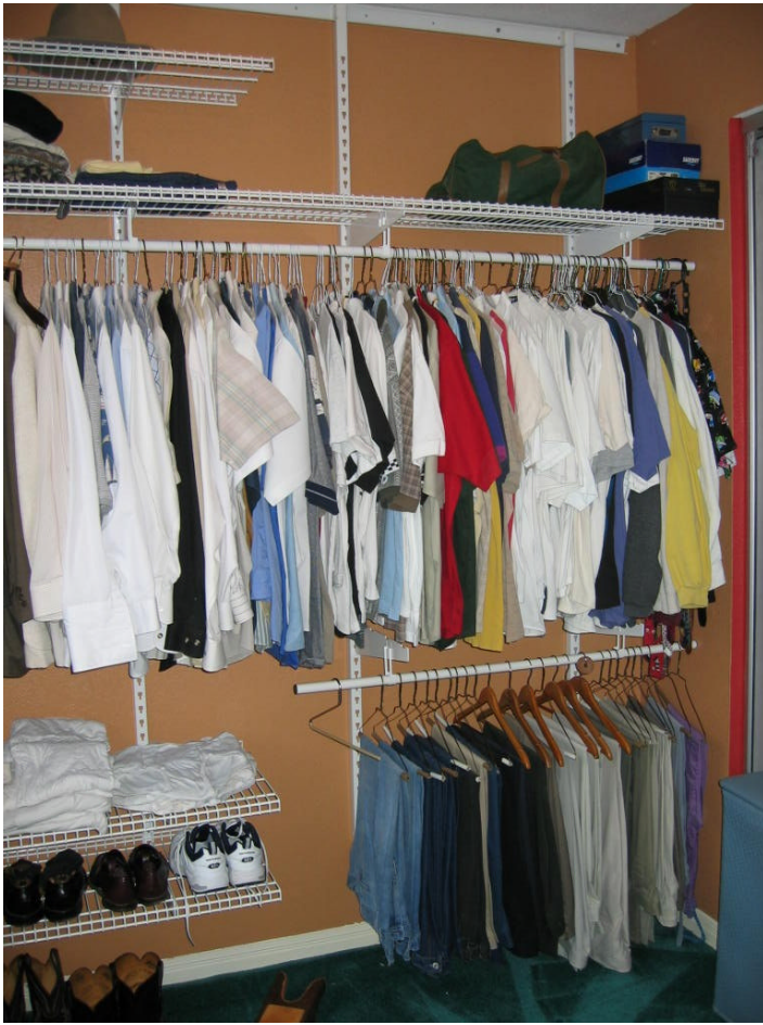
Short Wall trimmed 48" top rail, verticals & shelves adjusted to go around obstacles
